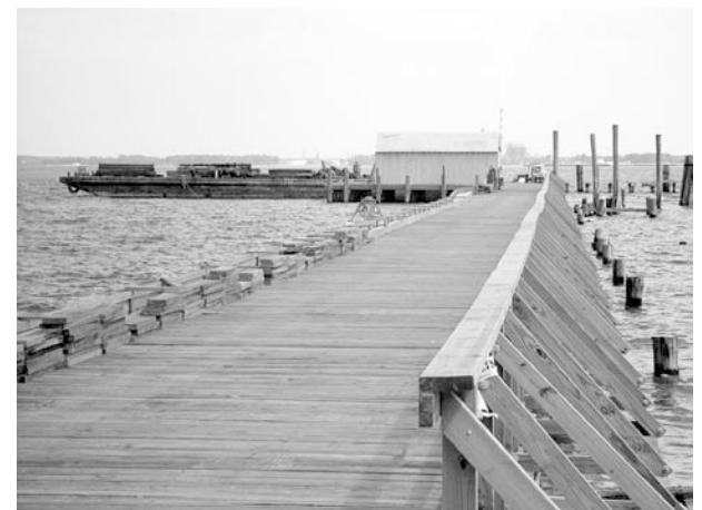
Construction crews have been using a barge-mounted crane to help rebuild the VIMS Ferry Pier, which was destroyed by Hurricane Isabel on September 18, 2003.
