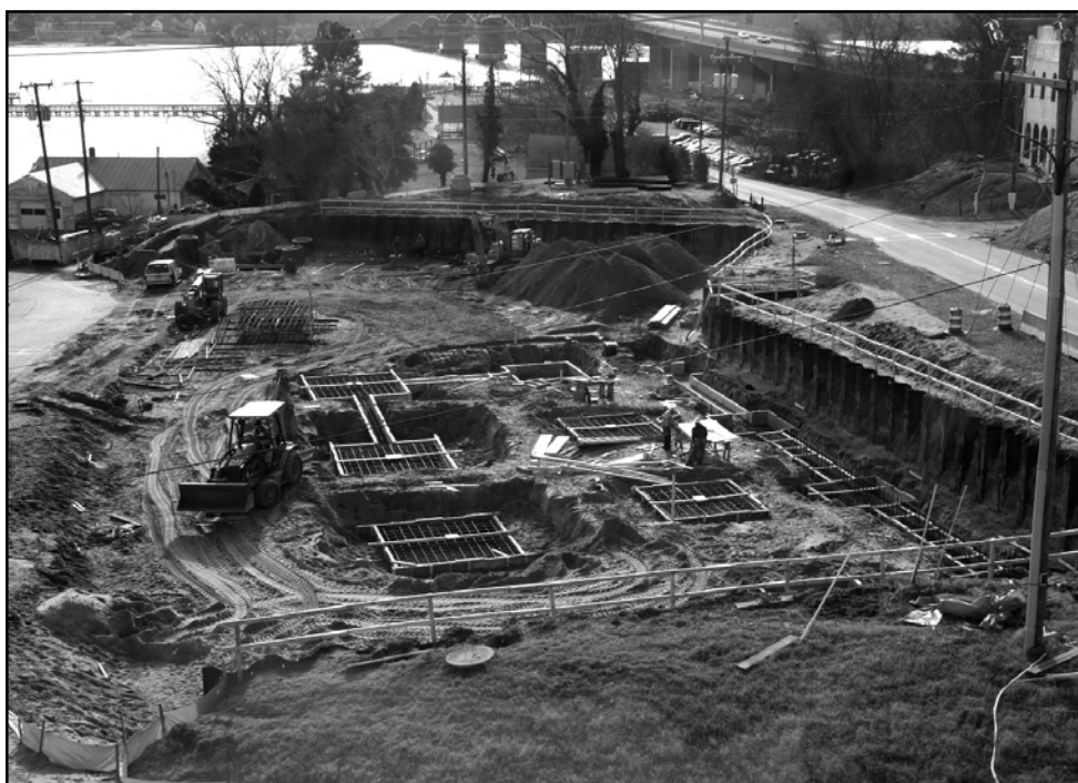
Workers prepare the footers to be poured for Andrews Hall.
