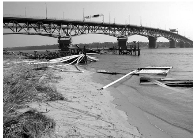
Remnants of pumphouse at the boat basin.
