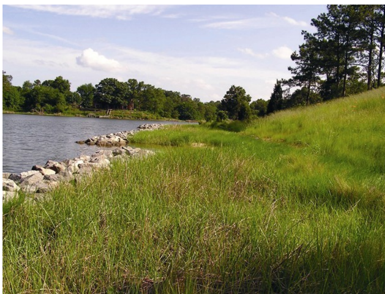
Figure 9.1. Example of a living shoreline installed as an alternative to an exclusive revetment erosion control structure. Photo credit: Karen Duhring.
