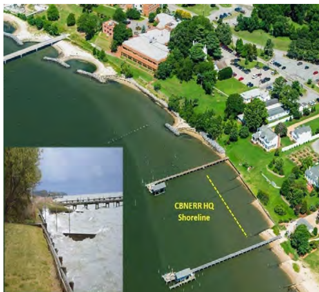
Figure 11.4. Aerial view of CBNERR-VA Headquarters highlighting location of failing shoreline protection infrastructure. Image sources: VIMS and W. Reay.
