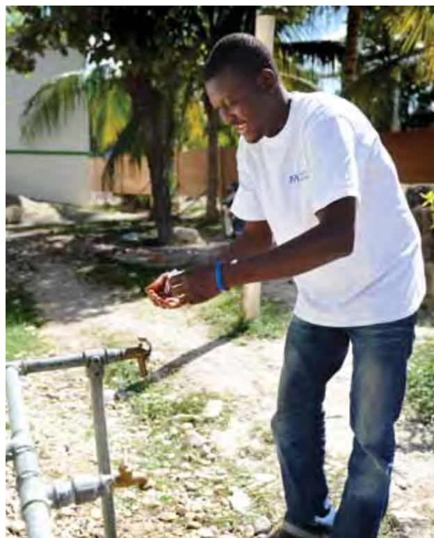
Checking the chlorine level of drinking water outside of Verrettes Hospital in Haiti.
