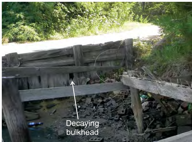
The bulkhead that supports the paved ramp leading to the dock is decaying and needs replaced.
