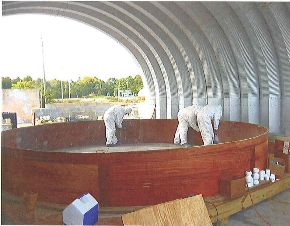
A wooden tank was constructed and then covered in fiberglass.
