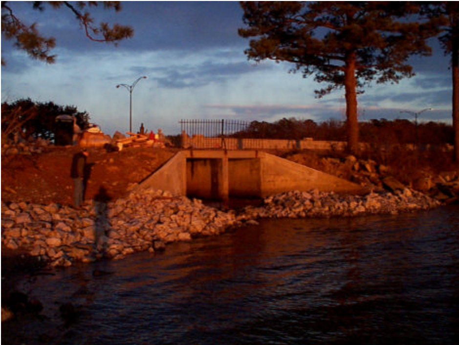
Figure 5. Outflow of Lake Maury spillway. Irish ramp was near head
