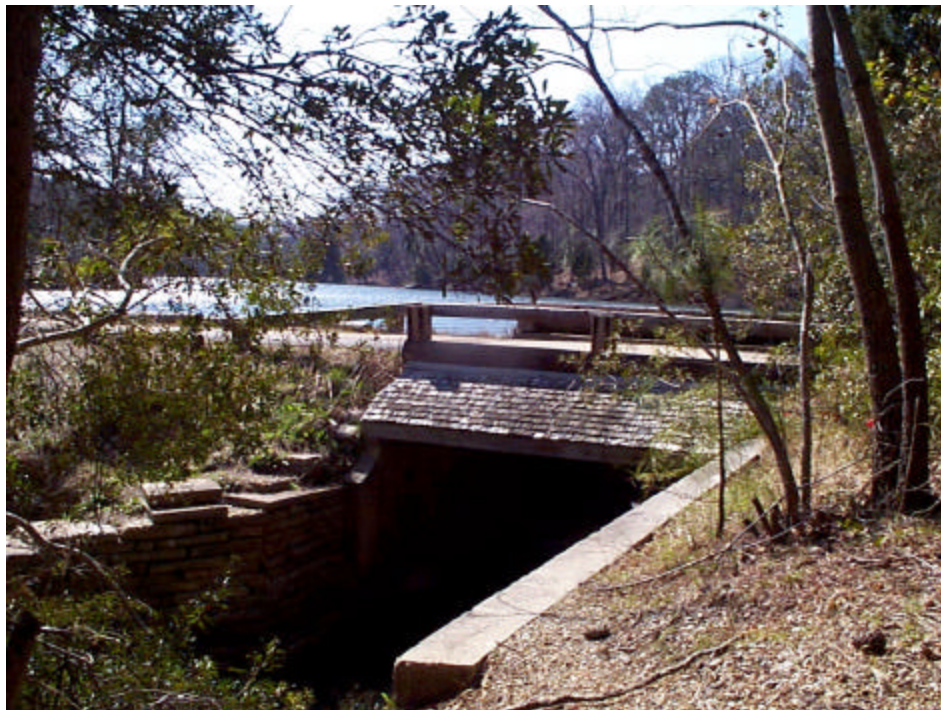
Figure 3. Bridge over Wormley Creek with Wormley Pond in background. Irish ramp was set under upstream edge of bridge at the base of the dam.
