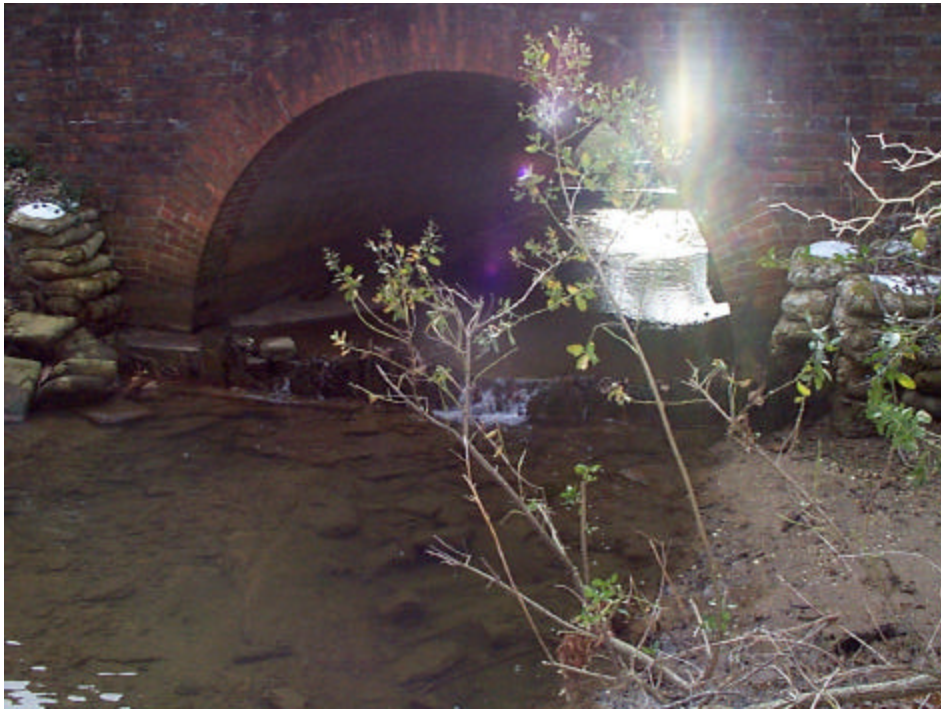
Figure 2. Brackens Pond spillway and tailrace. Irish ramp was set against the right wall on upstream end of culvert.
