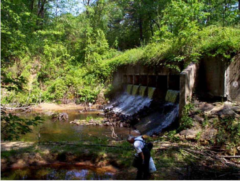
Figure 4. View of Kamp's Millpond spillway and tailrace.
