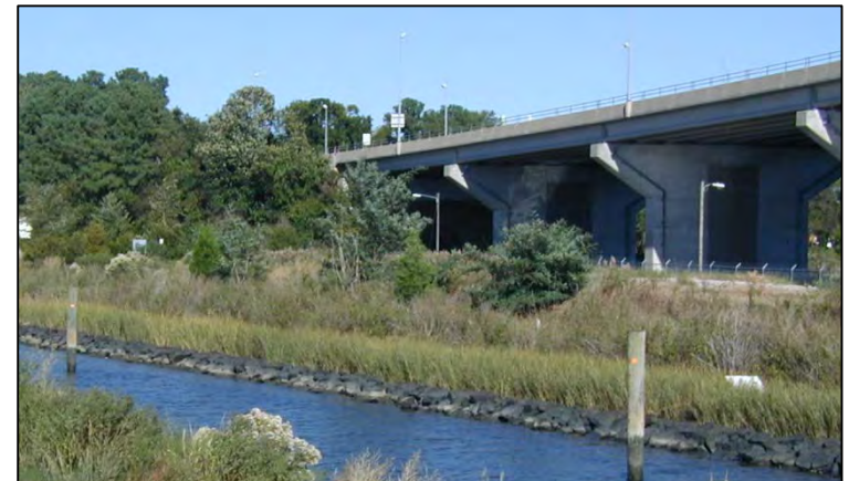
VIMS Marsh Sill constructed 1984
