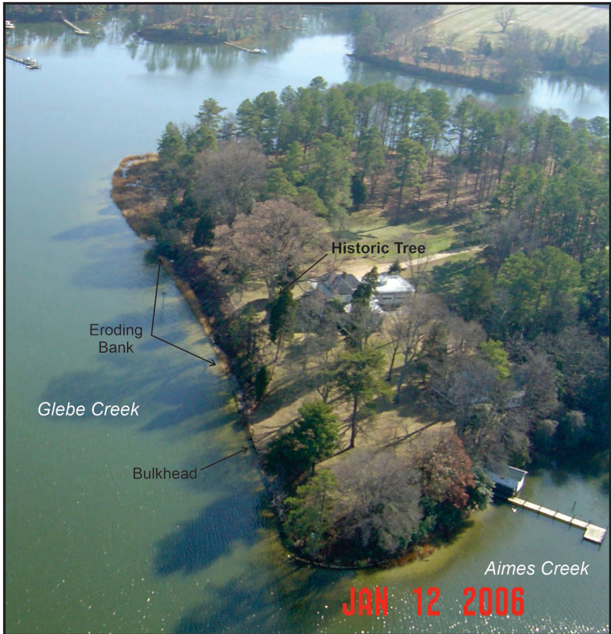
Figure 9-4. Aerial photo of the peninsula that Hull Springs Farm sits on. The shoreline has a high eroding bank and a failing bulkhead. The historic tree was a key part of the project design. Photo credit: Shoreline Studies Program, VIMS.
