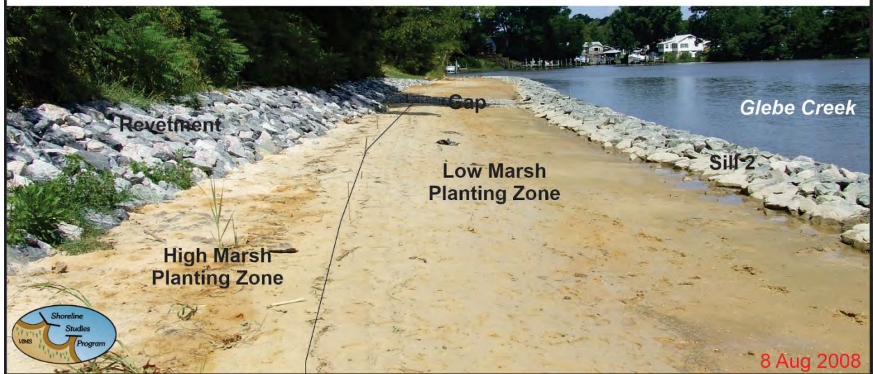
Figure 9-10. Post construction ground photos showing the low and high marsh planting zones. The marsh was planted soon after.
