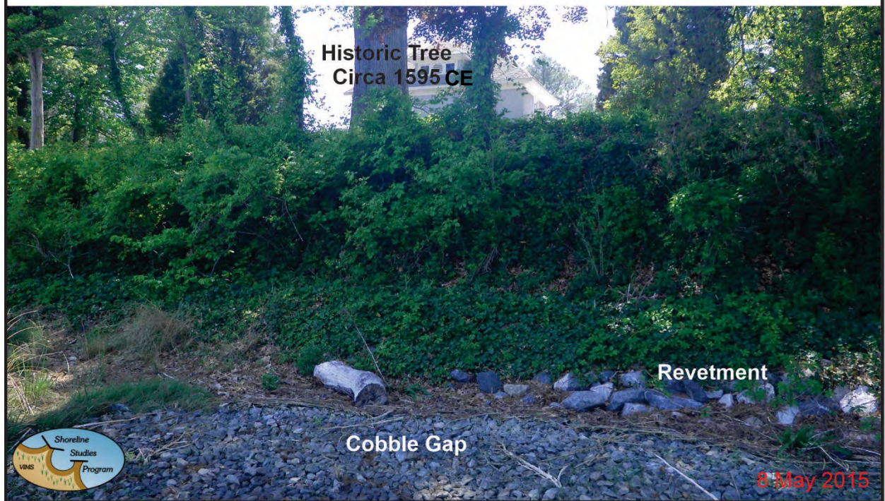
Figure 9-12. Hull Springs Farm about 6 years after construction. Top: Sill 2 has lush low marsh behind the structure, but the high marsh is not as vegetated. Bottom: The bank has slumped over the revetment. The sediment is vegetated which adds additional stability to the bank to protect the historic tree. Photo credit: Shoreline Studies Program, VIMS.
