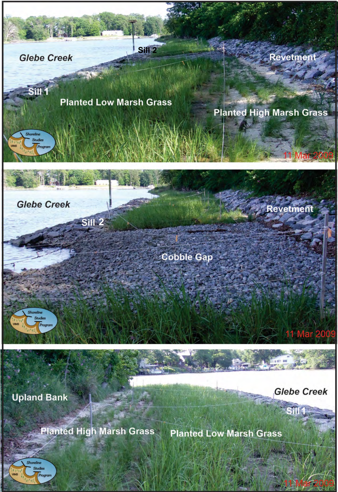
Figure 9-11. Hull Springs Farm living shoreline after about 1 year. The elements were constructed as designed, and the low marsh has filled in well. Photo credit: Shoreline Studies Program, VIMS.
